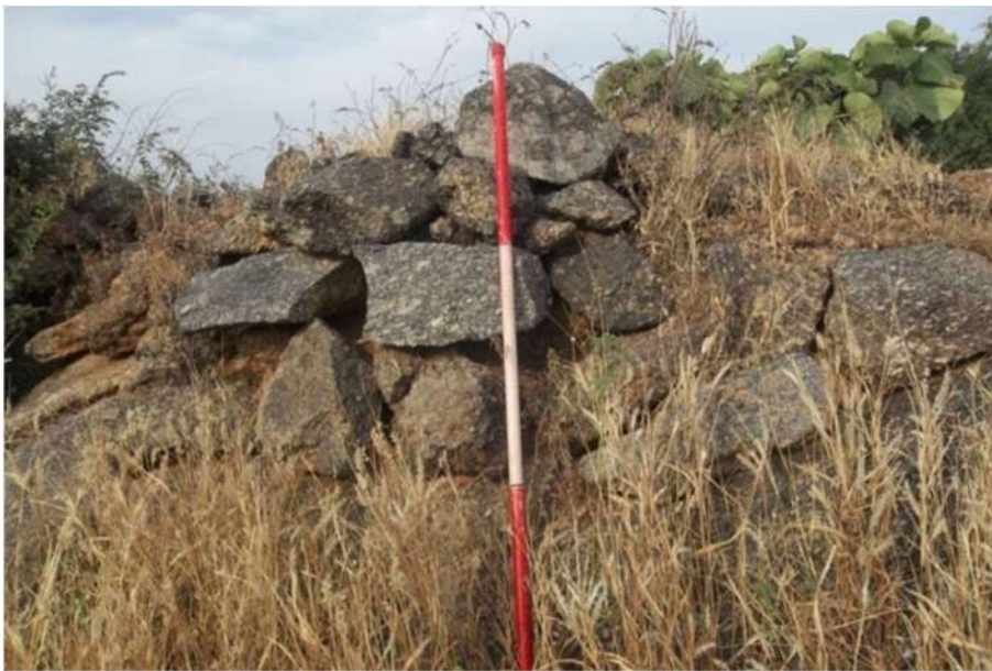
Plate 6: Defensive wall at Kurkutawa site
