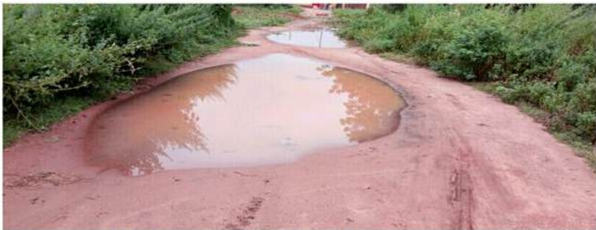
Plate Ib: An Example of Water Ponding in Concavities Along Untarred Roads
