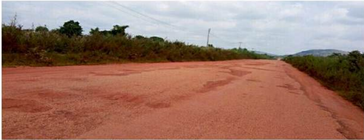
Plate Ia: A Degraded Road in the Study Area Without Man-made Drainages.
